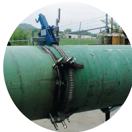
Dearman Light Double Jackscrew Chain Clamp aligning 24" Schedule 40 pipe prior to welding.
